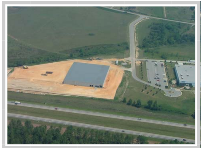
Steeplechase Shell Building #3
